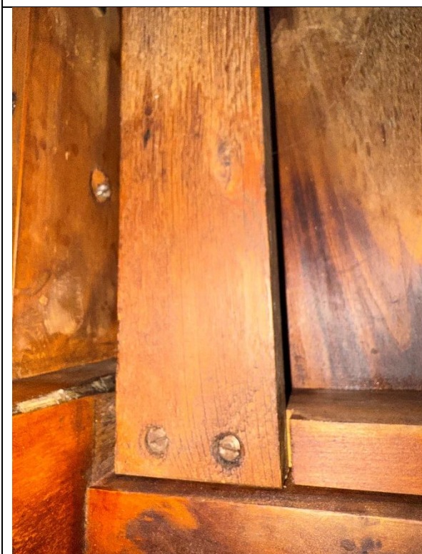
Figure 3: Machine-cut Flathead Screws
